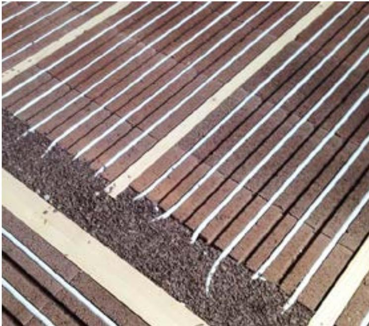
*The perfect combination: heating coils and moulded tiles from Lithotherm in combination with the Cemwood CW 2000 fill*
